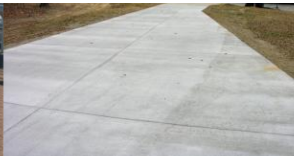
General campus paving Standard gray concrete, light broom finish Concrete to contain minimum 15% slag, 15% fly ash to meet LEED standards.
