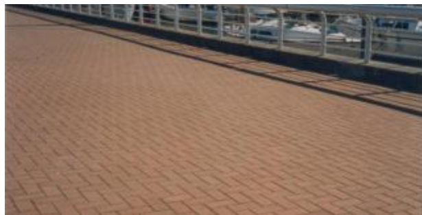
Pacific Interlock Pavingstone Etchable Donor Pavers Holland Classic paver. Paver color to have SRI of 29 or above.
