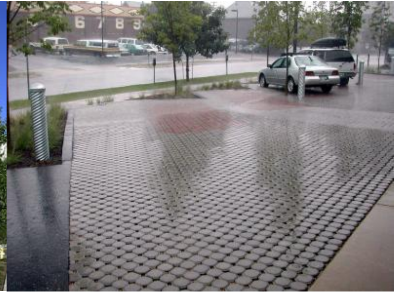
Pacific Interlock Pavingstone Hydro-Flo Permeable Pavers Paver color to have SRI of 29 or above.
