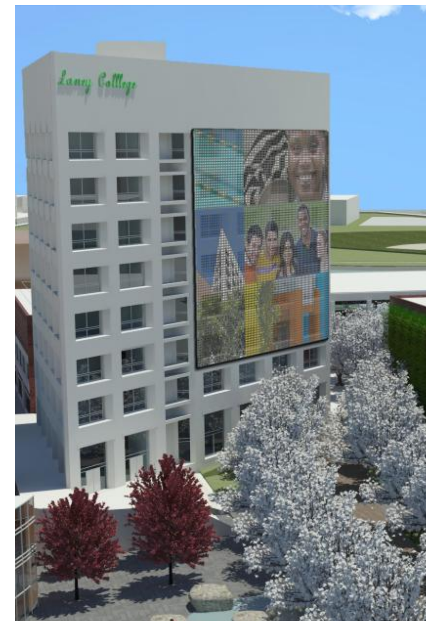
MESH SCREEN ON TOWER ADMINISTRATION
