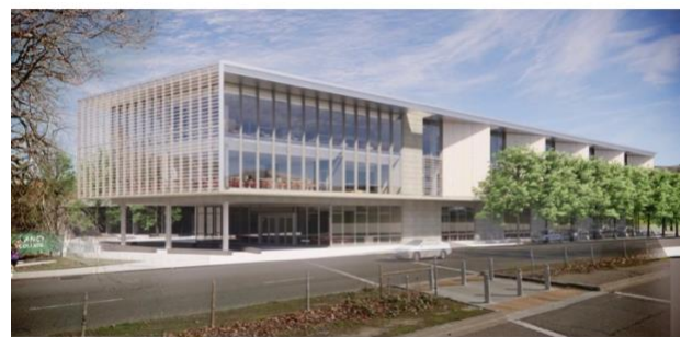
PROPOSED LIBRARY / LRC ALONG 7 TH STREET P000 LANEY COLLEGE LIBRARY & LRC CD PROGRESS UPDATE | OCTOBER 16, 2020 Laney College: visualization of new Learning Resource Center
