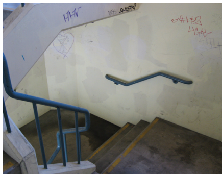
Building G South stair
