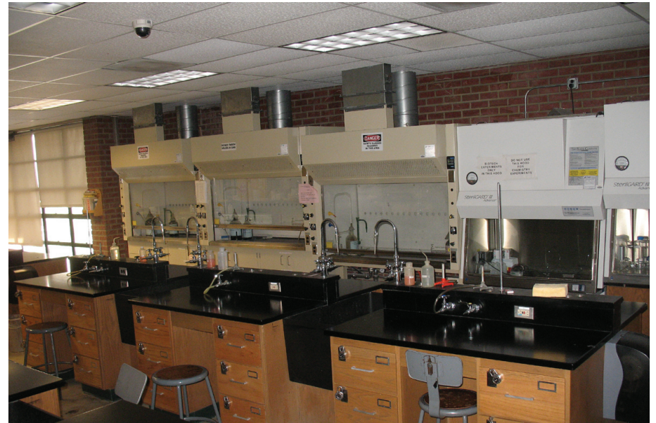
Typical existing science lab
