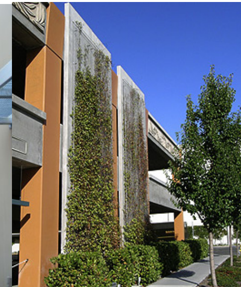
Greenscreen Trellis screens Galvanized steel, powder coated.
