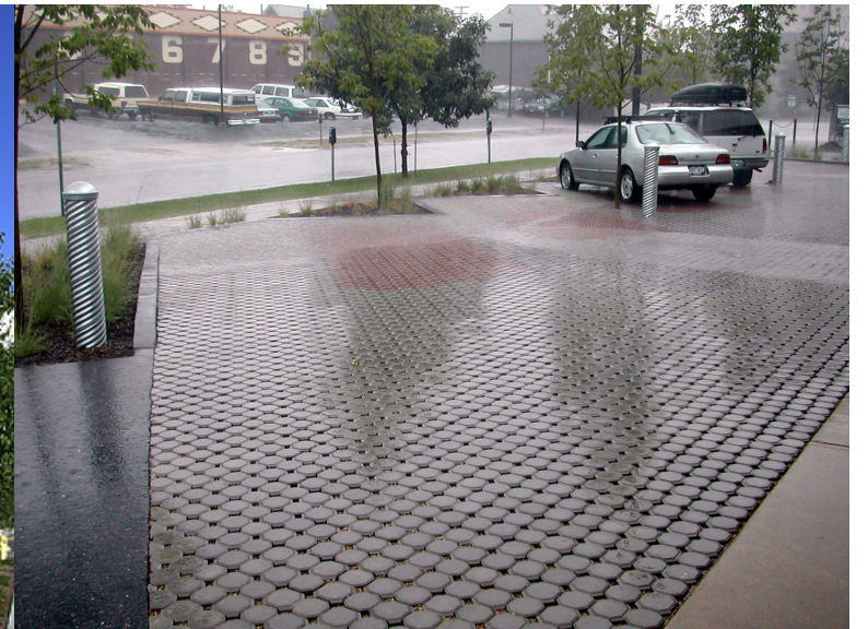
Pacific Interlock Pavingstone Hydro-Flo Permeable Pavers Paver color to have SRI of 29 or above.
