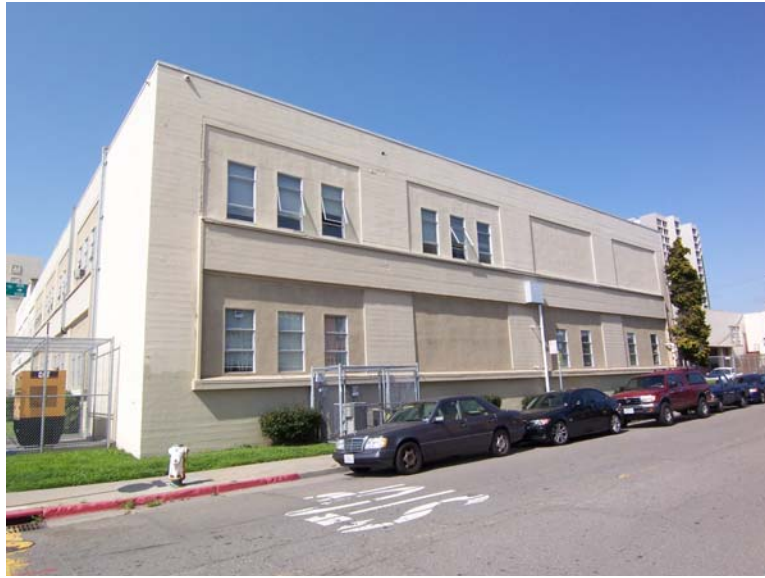
Figure 11. Southeast façade, March 2010 Source: KVP Consulting
