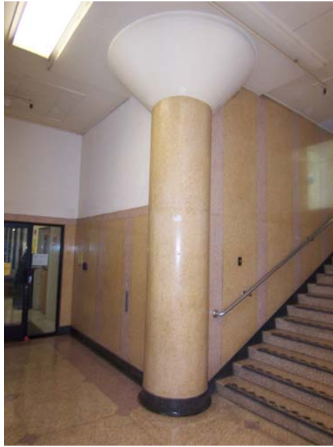
Figure 13. Detail of lobby, showing floor, column, and stairs, March 2010 Source: KVP Consulting
