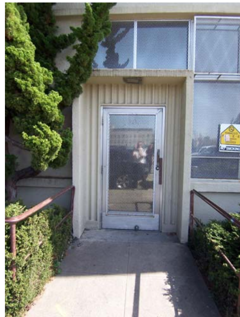
Figure 11. Pedestrian entrance on north façade, March 2010 Source: KVP Consulting
