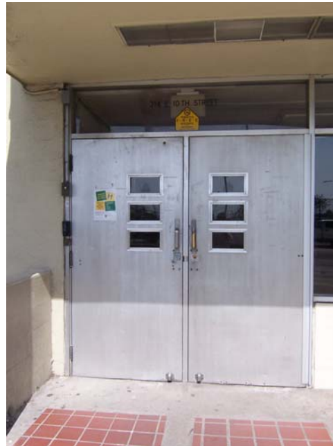
Figure 8. Main entrance, March 2010 Source: KVP Consulting
