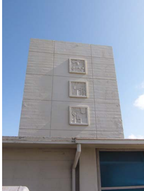
Figure 6. Sculptures on tower, March 2010 Source: KVP Consulting
