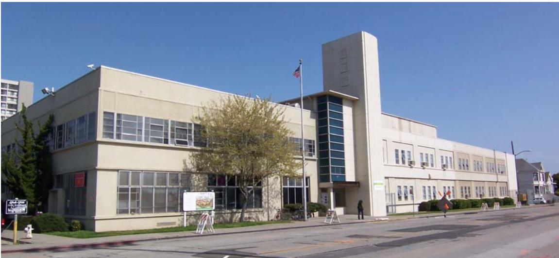
Figure 3. Main building, west façade, March 2010 Source: KVP Consulting
