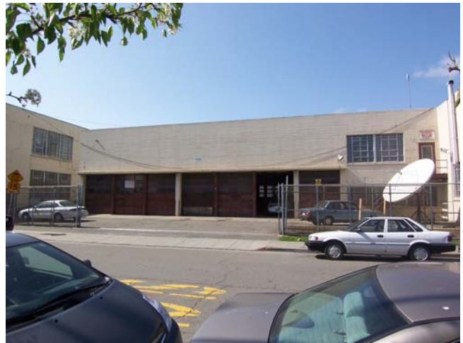
Figure 16. Southeast façade (southwest wing), March 2010 Source: KVP Consulting
