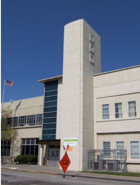
Figure 5. Stair tower, March 2010 Source: KVP Consulting
