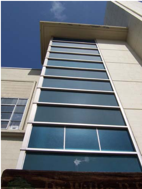
Figure 7. Stair tower detail, March 2010 Source: KVP Consulting
