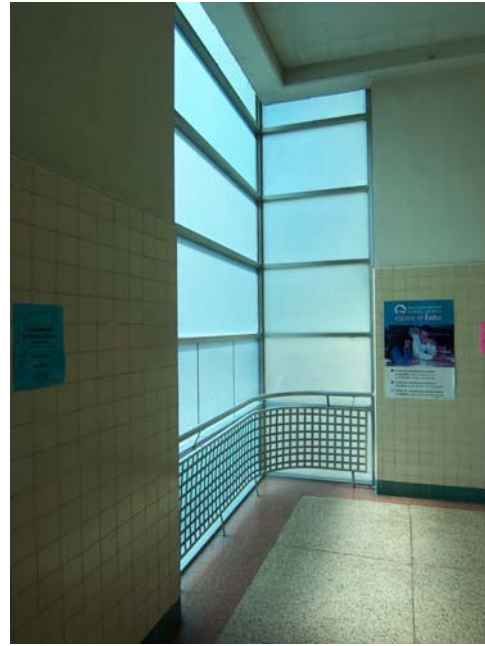
Figure 14. Interior of stair tower, March 2010 Source: KVP Consulting
